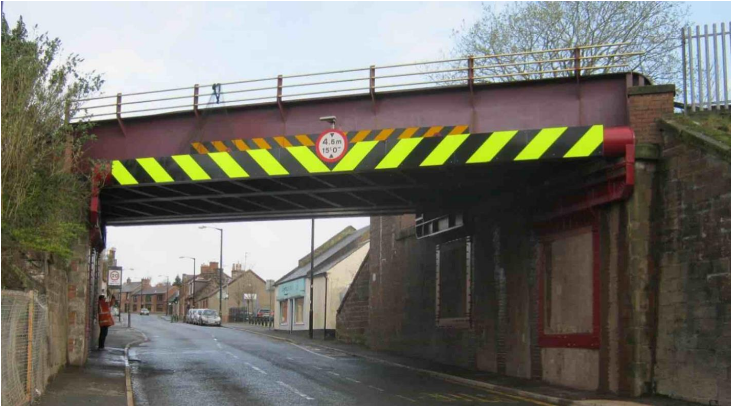
A Collision Protection Beam installed on a bridge. Photo Credit: Network Rail
