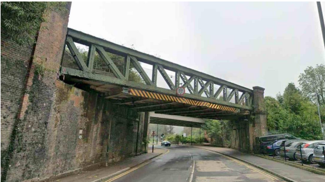
Coulsdon South Bridge, whereunder a truck, oops, “lorry” got stuck for half a day. The bridge is now to receive Collision Protection Beams. Photo credit: Network Rail
