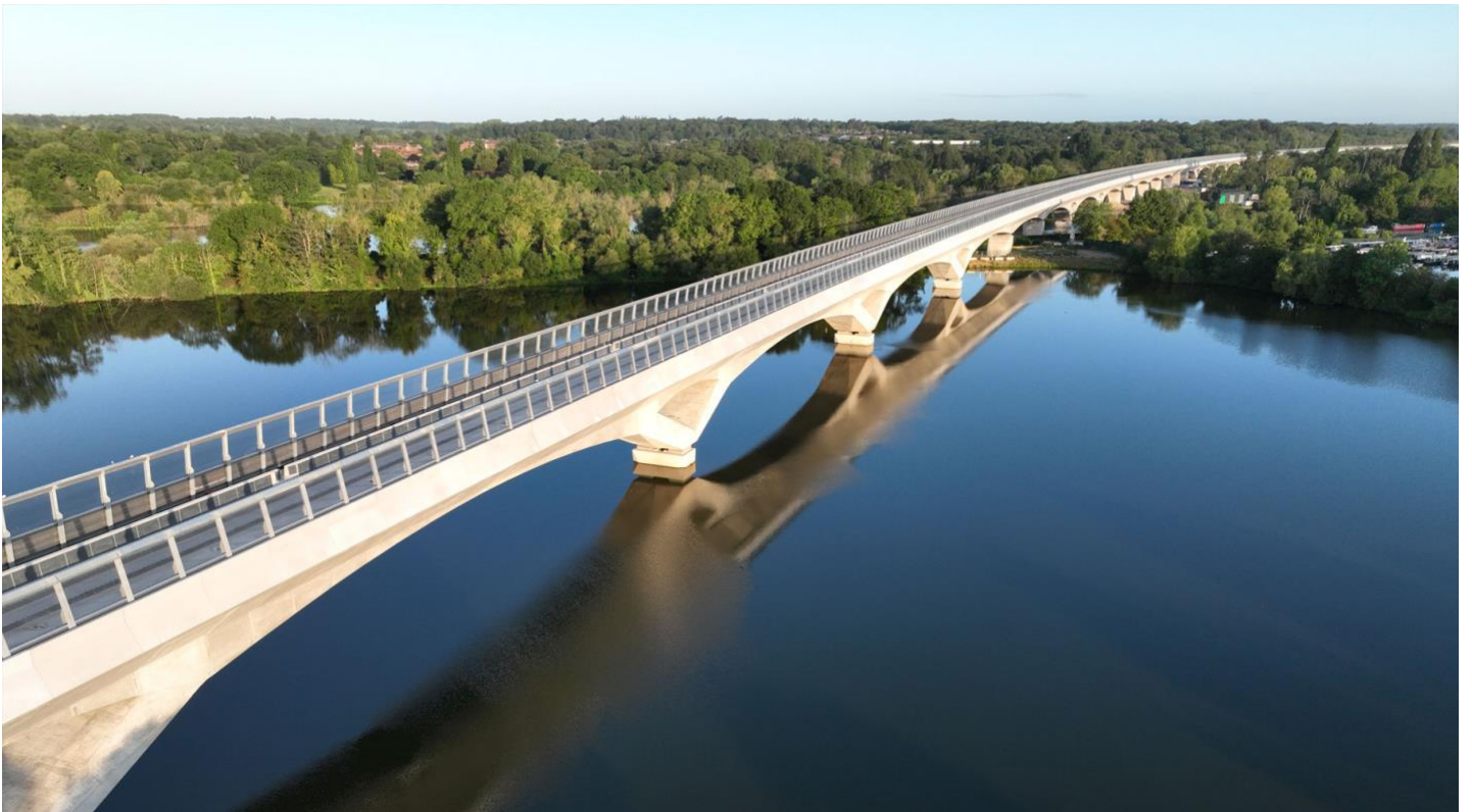
A drone's-eye view of the Colne Valley Viaduct.
